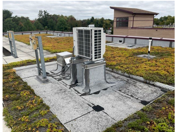
22 - SPLIT SYSTEM DUCTLESS
